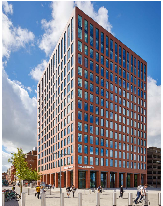
Thames Tower, Reading
